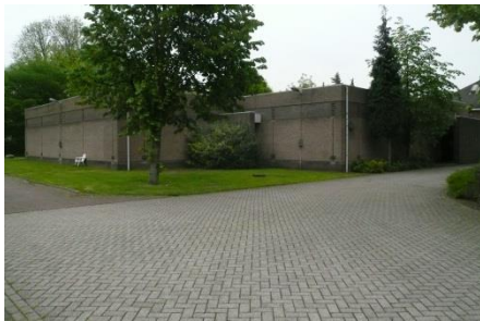
The bunker's exterior was camouflaged by using bricks
