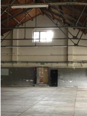
Interior of the Drill hall
